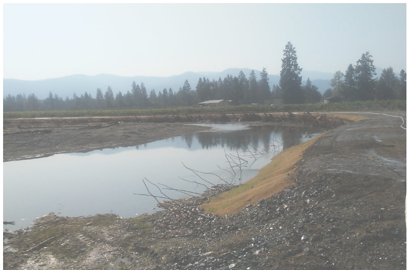
Above: Before bank stabilization at Bridgeview Vineyards. Below: After installation of woody structure, seeding and bank shaping.
