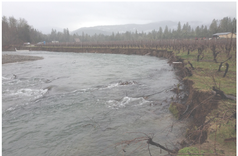
Above: Before bank stabilization at Bridgeview Vineyards. Below: After installation of woody structure, seeding and bank shaping.
