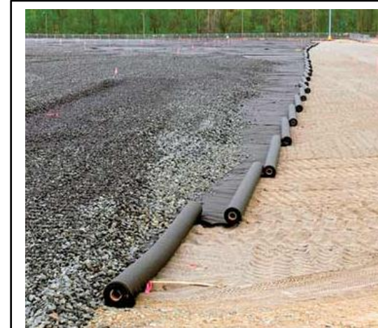
Left: Geotextile fabric is unrolled underneath gravel footing. Above: EcoGrid, a plastic footing grid
